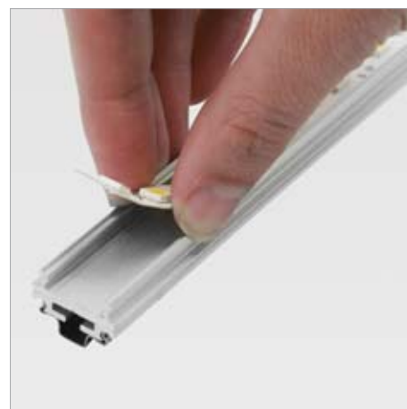
Remove the application tape from LEDtape and apply to Base
